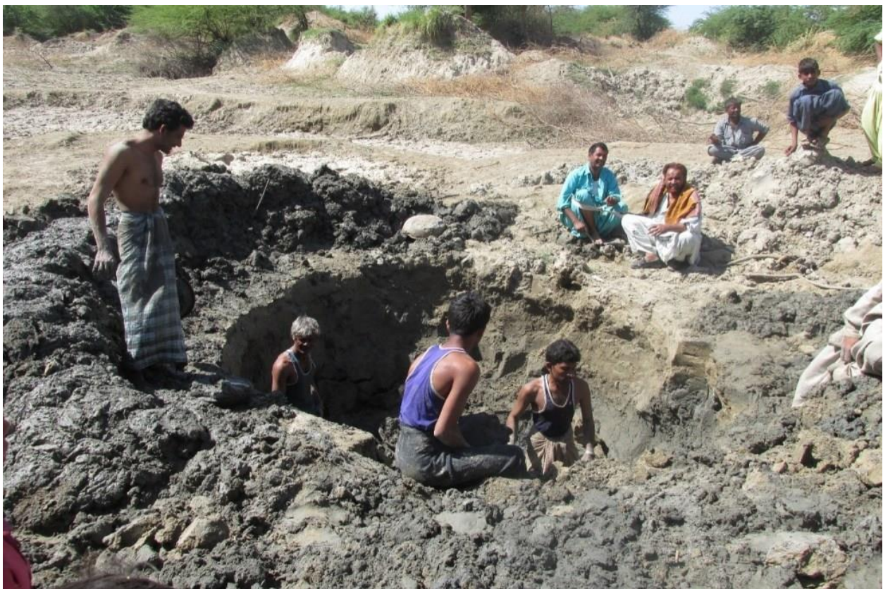
Photo Showing People Digging The Soil In Search Of Water At Kutch
